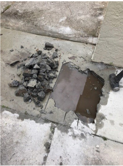
Figure 5 – Brown Muddy Water Quickly Filled the Concrete Excavation
