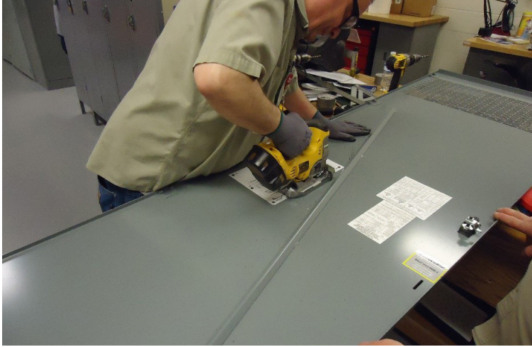
Figure 1 Field Installation of IR windows using provided Templates and a Jigsaw
