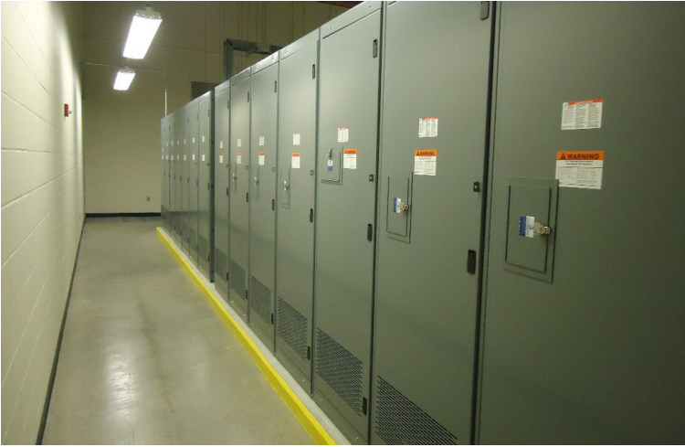
Figure 3 Finished Installation of CAP-CT-12 Infrared Windows
